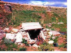
This photo shows the end of the shelter next to the entrance. Note the 4 foot diameter culvert coming off the left just before the bed. The entrance pipe wasn't put on the very end of the 50 foot long culvert for a very good reason - so the bed would fit. Note also the vent pipe in the ceiling. The owner said he would cut it off close to flush with the ceiling if he had to do it over again.
