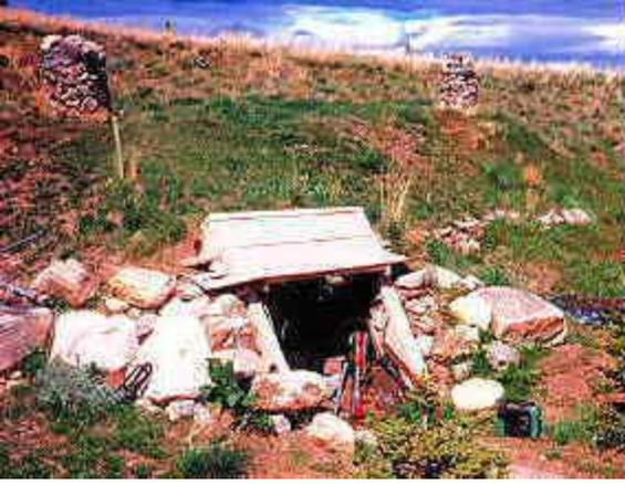
This photo shows the end of the shelter next to the entrance. Note the 4 foot diameter culvert coming off the left just before the bed. The entrance pipe wasn't put on the very end of the 50 foot long culvert for a very good reason - so the bed would fit. Note also the vent pipe in the ceiling. The owner said he would cut it off close to flush with the ceiling if he had to do it over again.
